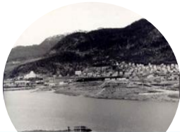
Start construction Mosal
