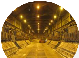
Extension Prebake Line 2
