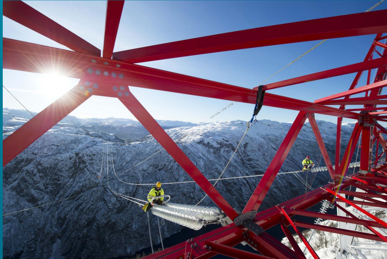
Picture: Work on power line.
